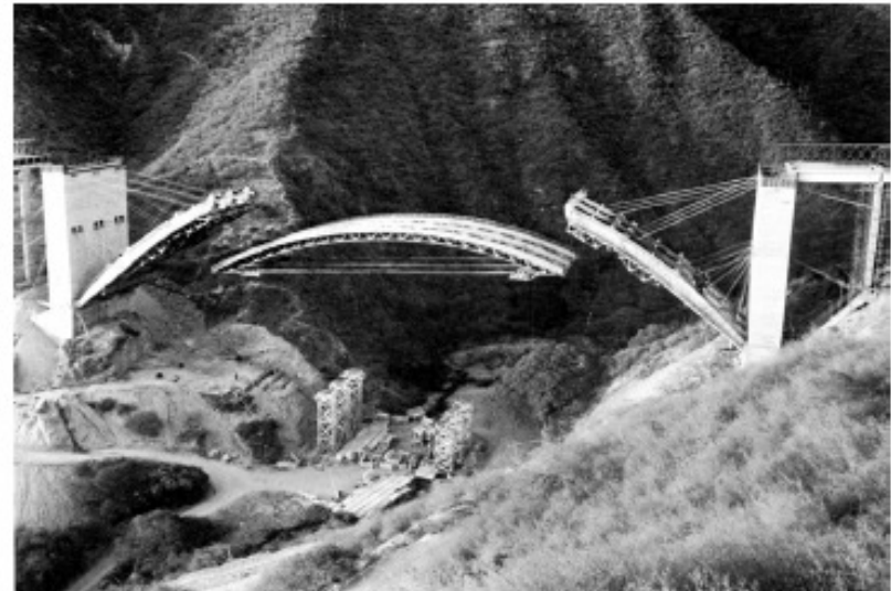
Figure 21 - Caracas Viaduct during construction
